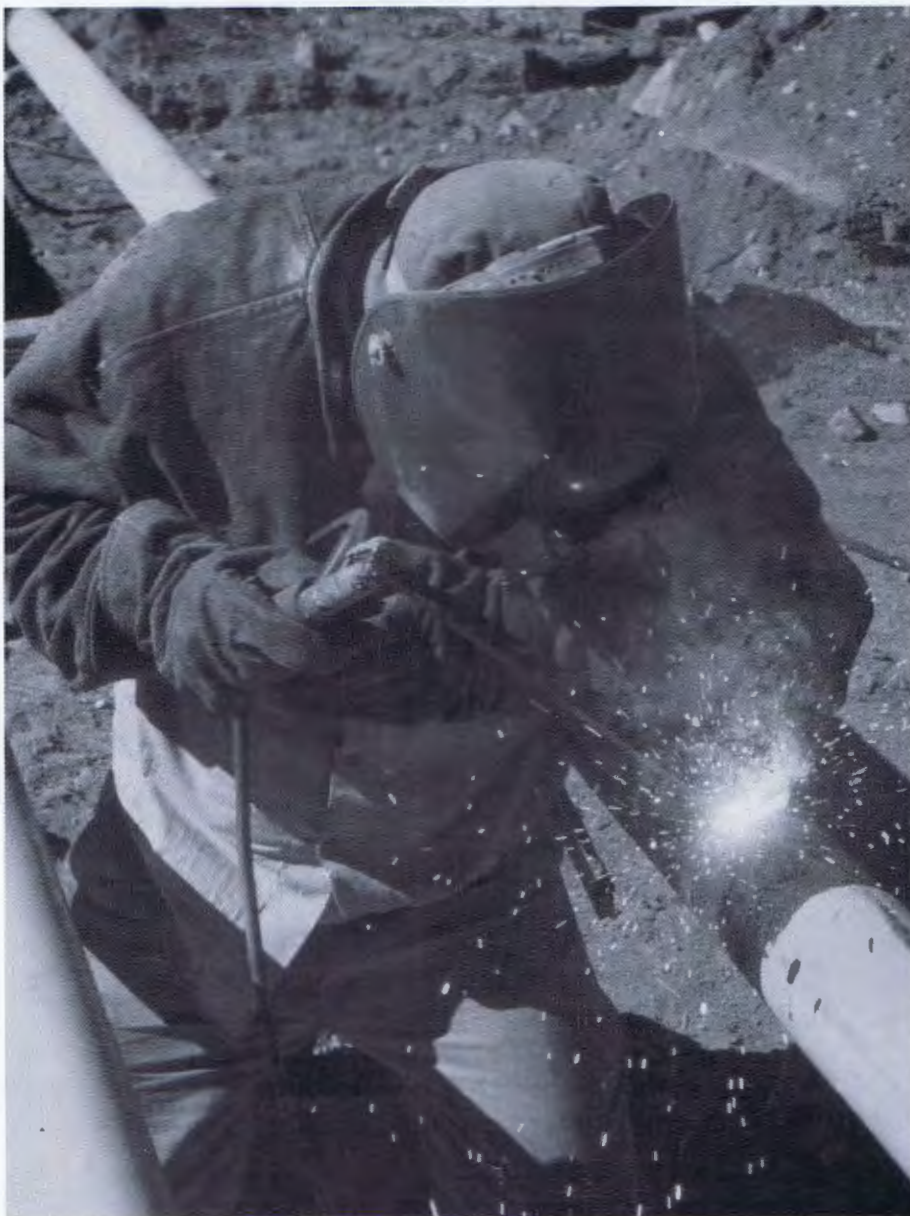
A Southwest Gas employee welds new pipeline.
